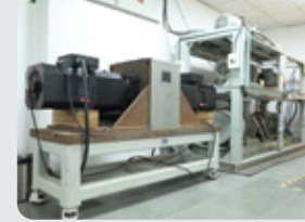
POWER ELECTRONICS DESIGN CENTER
