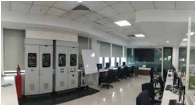
Manufacturing Design Centre, Bengaluru
